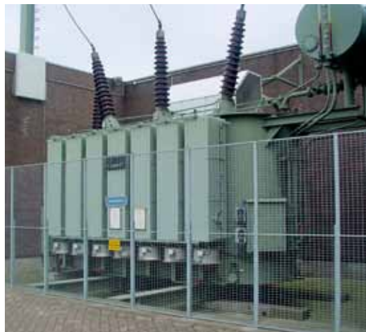
HS/MS-transformator
