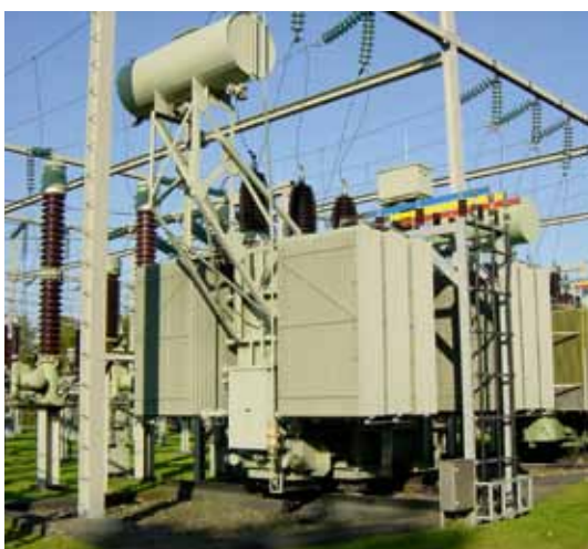
HS/MS-transformator
